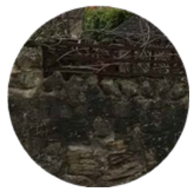
Stone boundary wall
