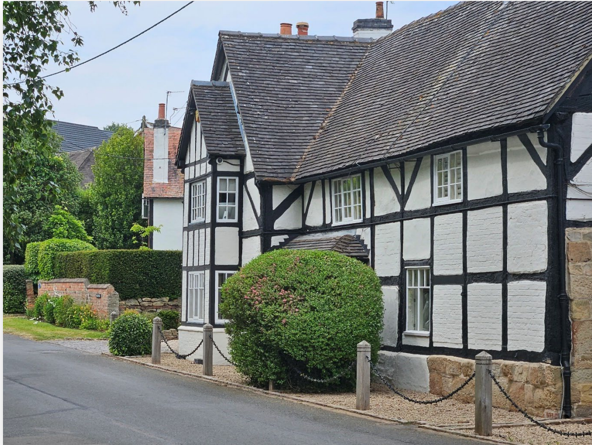
Figure 13: Brook House, Wilson
