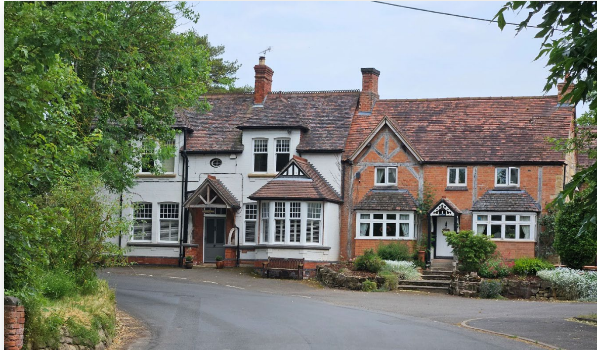
Figure 17: Wilson Conservation Area
